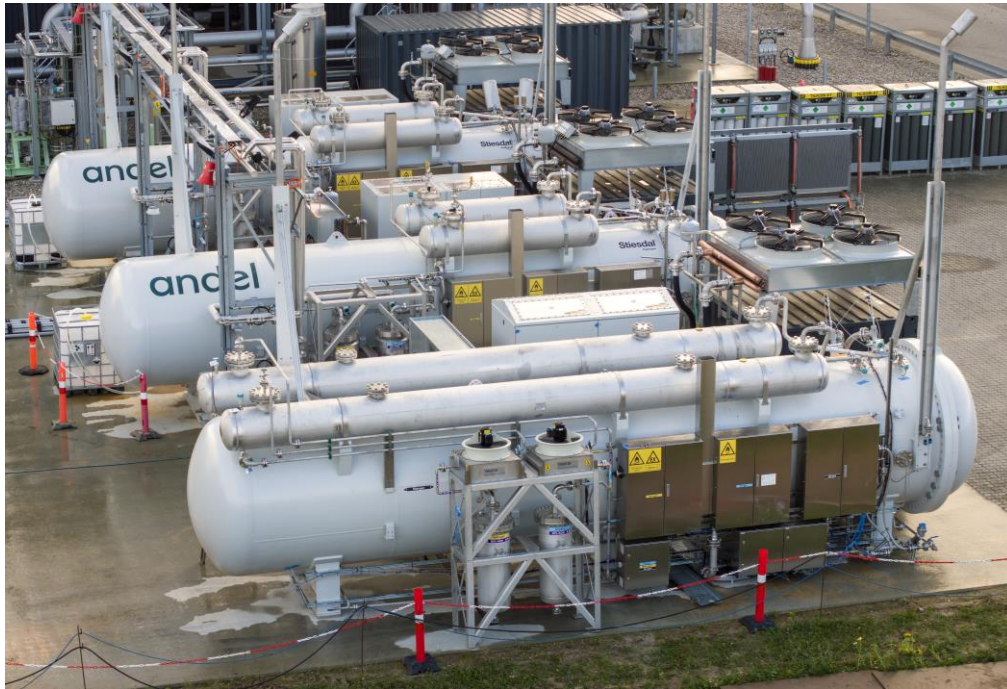
Glansager Biomethanisation Plant (DK) Three Electrolyzer Units
