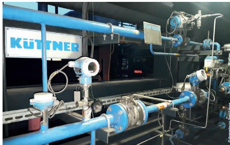
Valve station at blast furnace with vortex flowmeter plus pressure and temperature compensation for hydrogen measurement.
