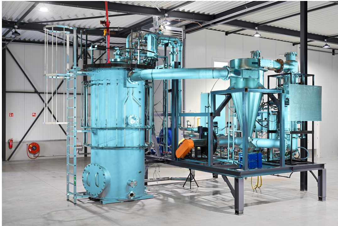
Combustion research by Iron+ at Metalot Future Energy Lab, 200 kW
